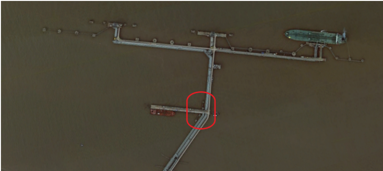
Figure 1 Structure between end of IOT Finger Pier Berths 7 and 9 and IOT trunkway
